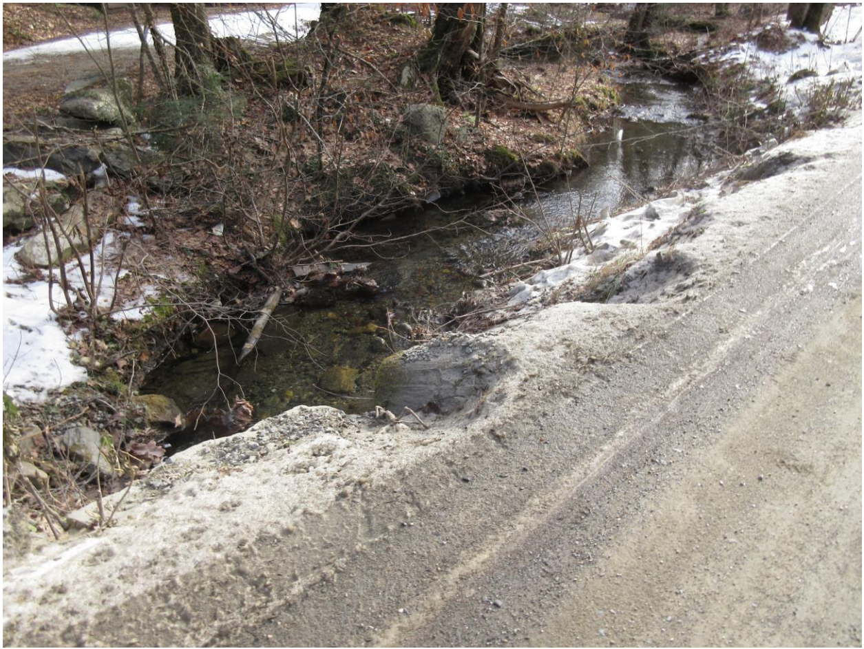
Outlet and bank erosion (Above and Below)
