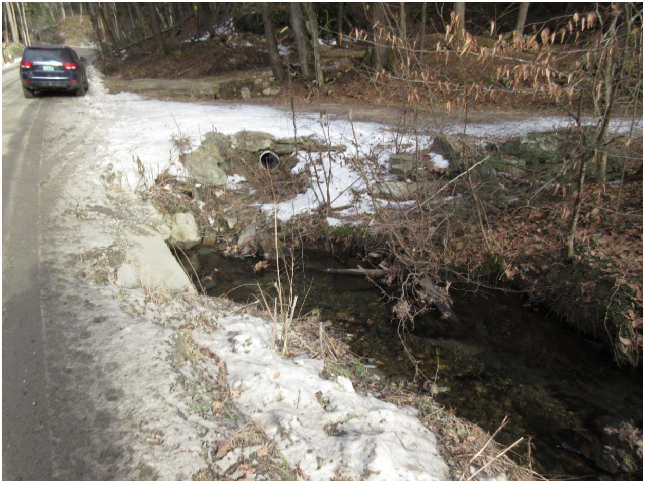
Outlet and bank erosion (Above and Below)
